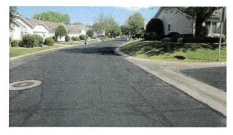
Most asphalt areas can be expected to last approximately 30 to 40 years before it will become necessary for an overlay to be applied. It will be necessary to adjust manhole and valve covers at the time the overlay is applied. Deflection testing should be conducted by an independent consultant near the end of the estimated useful life to determine the condition of the asphalt and estimated remaining life before the overlay is required.
