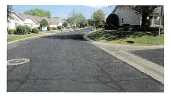
A type II slurry seal or seal coat should be completed every 6 years so that the life of the asphalt will be extended. We have budgeted this for 2023. 51,620 sq. ft.
