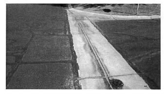
This is for the cleaning and sealing of cracks. We have budgeted to have this completed every 3 years beginning in 2023. We have budgeted for repairs which includes surface patch, crack repair and asphalt joint seal. This component is important in that it will extend the life of the asphalt if it is completed in a timely manner.
